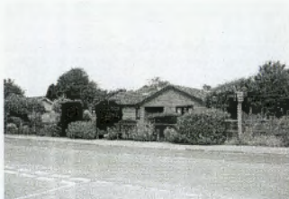
Station Road Black Fascias & Bargeboards
